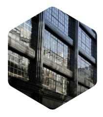
Carefully crafted iridescent blue-glazed Faience tiles, frame steel Crittal Windows, shuttered concrete soffits, curtain wall glazing and clay-engineering bricks have been brought together by this Master Builder to create an incredible new landmark office built to stand the test of time.
